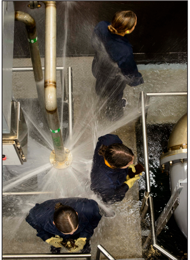
Midshipmen practice properly repairing a water pipe using a strong back patch at the Trident Training Facility onboard Naval Submarine Base Kings Bay, Georgia.
