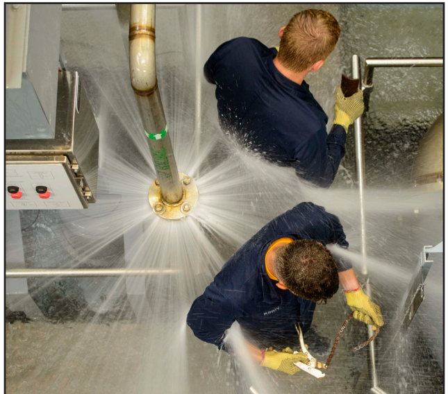
Midshipmen practice properly repairing a water pipe using a strong back patch at the Trident Training Facility onboard Naval Submarine Base Kings Bay, Georgia.
